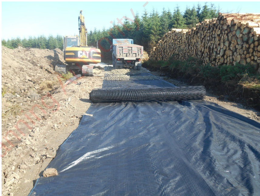
Figure 15: Access Track Build-up with Geotextile
