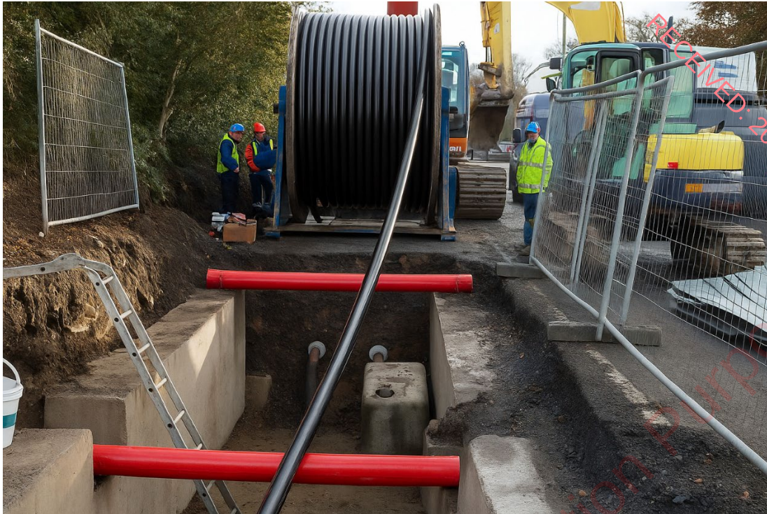
Figure 13: HV cable pulling procedure (Typical drum set-up)
