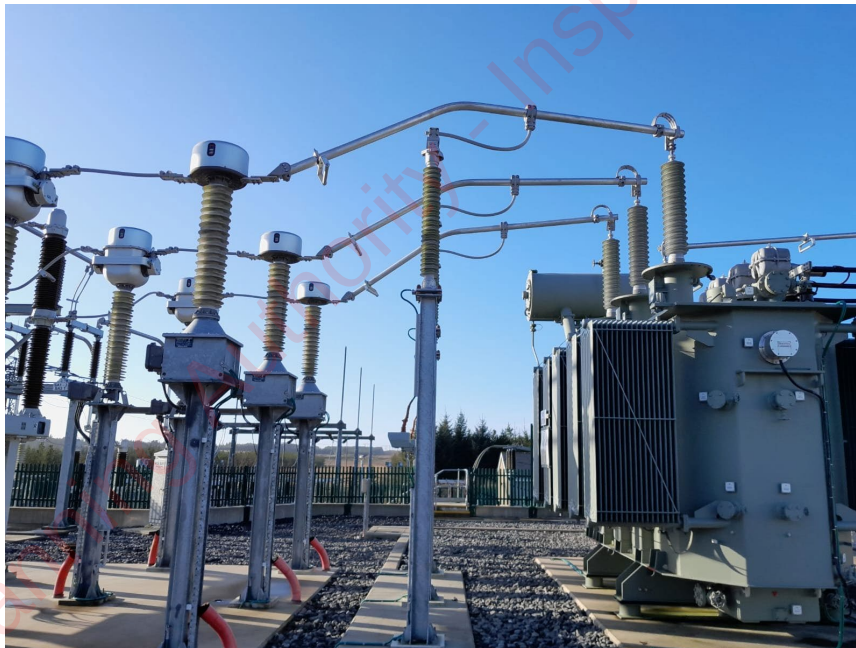
Figure 8: Typical 110kV Transformer Connection
