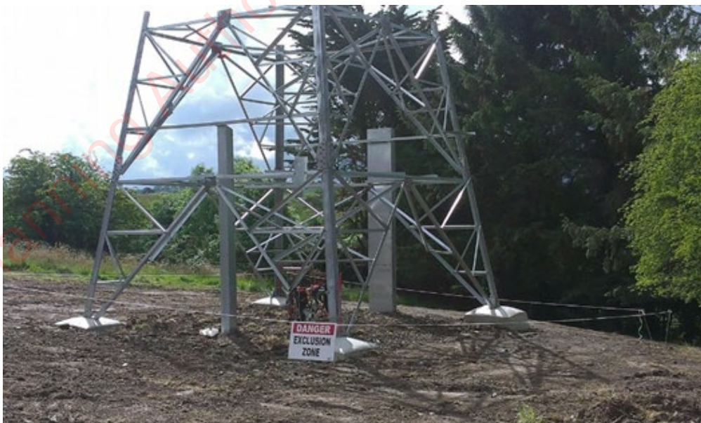
Figure 4: Base of End masts Structure Backfilled
