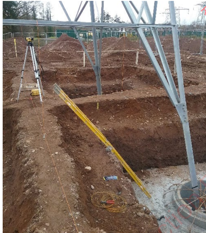
Figure 3: Typical 110kV end masts foundation excavation
