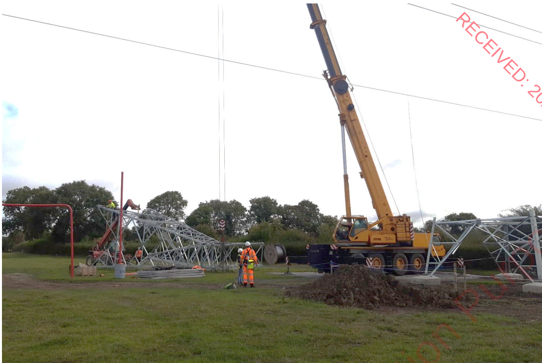
Figure 16: Crane pad and laydown areas
